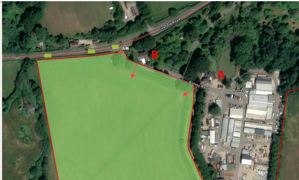
Above: Aerial photograph of properties A: 'The White House' and B: the 'adjacent property' and the Oakendene West construction compound shown in green to the south of the A272. Screenshot capture taken from Rampion 2 WSP WebGIS platform, showing scheme information also displayed within Landscape elements Figure 18.8t, Aerial imagery source: Esri, Maxar, Earthstar Geographics, and the GIS User Community 2023.
